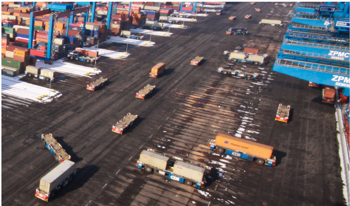
Illustration 1: ©Frank Grunwald, Picture from the top of one of the container bridges of the HHLA Container Terminal Altenwerder (CTA) in Hamburg. You can see the Blocklager and the AGVs.
